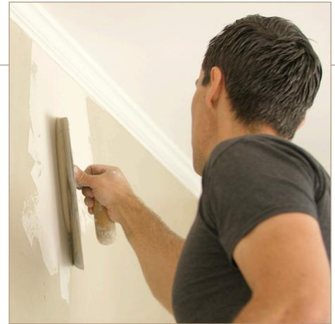
Applying the second thin coat of LSB Interior Finish over drywall.
