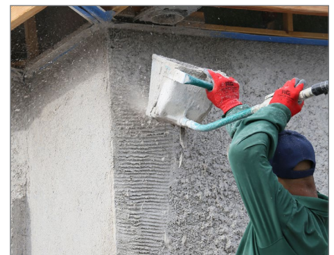
FIG 09 - Spray-applying LSB Binder leveling coat over keyed scratch coat.
